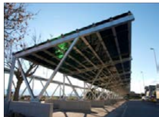
Figure 7. Photovoltaic Parking Lot Design and real project in Lamezia Terme, Italy. Source: Onyx Solar.
