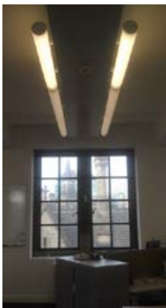
Figure 5. Typical Lighting Pod in the THX Office Floors.
