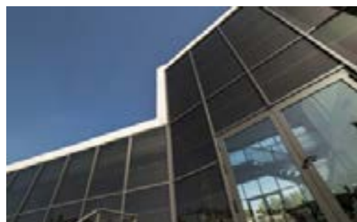
Figure 3. PV Curtain Wall scheme and real integration in Guadalhorce Headquarters, Málaga (Spain). Source: Onyx Solar.
